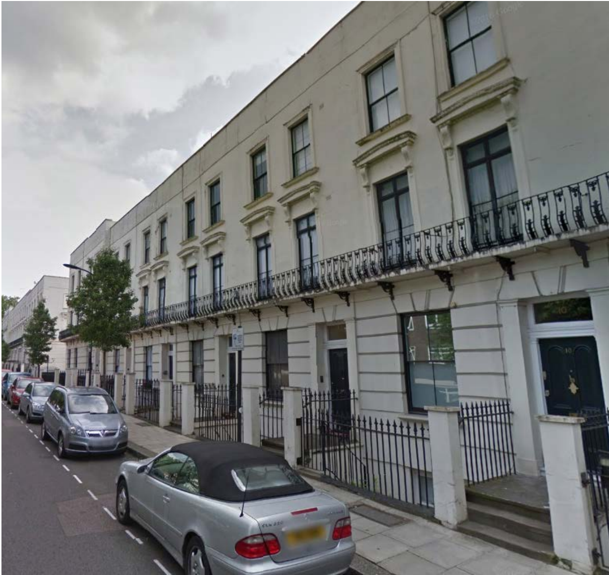
Front elevation of Nos.12-14 Blomfield Villas.
