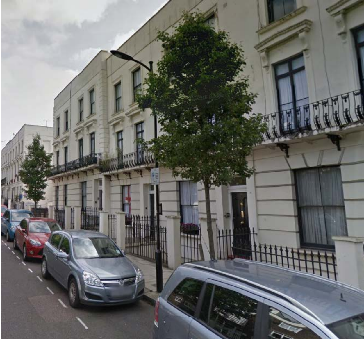
Front elevation of Nos.16-18 Blomfield Villas.
