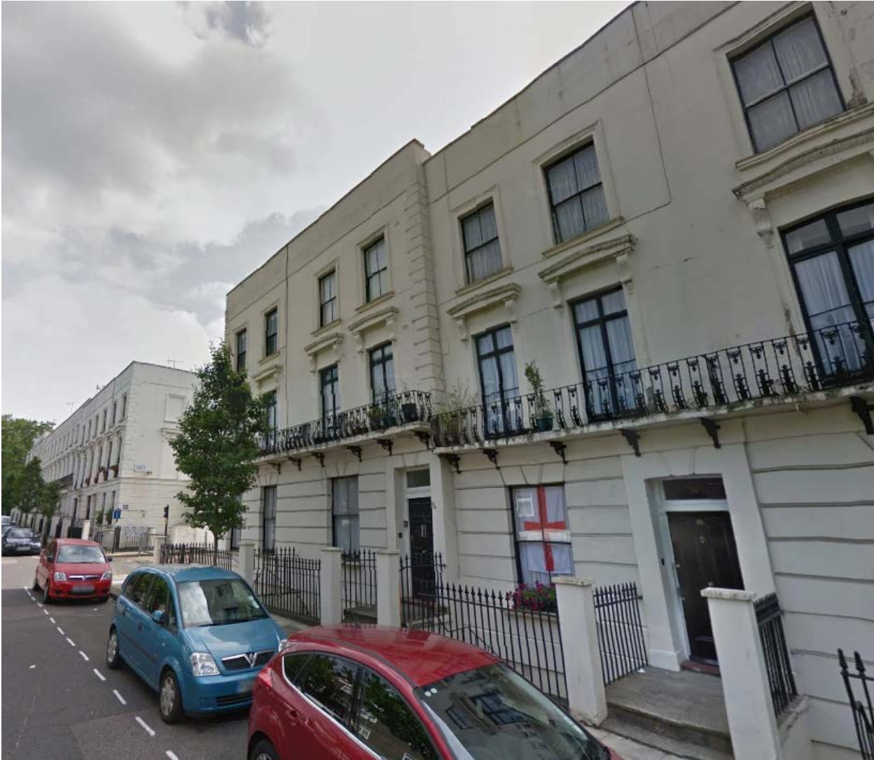
Front elevation of Nos.20-22 Blomfield Villas.
