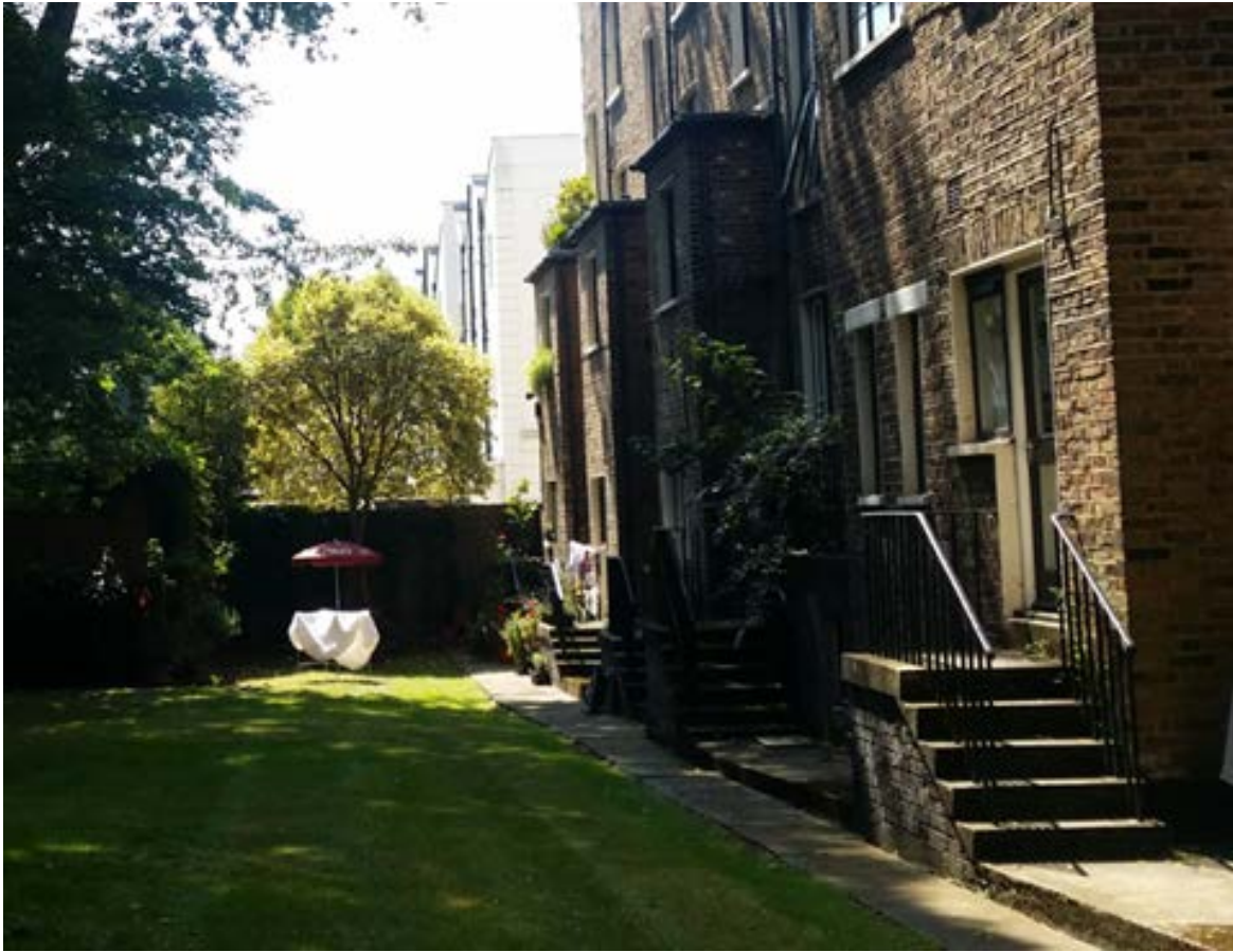
Rear elevation of Nos.24-46 Blomfield Villas in context with communal gardens.
